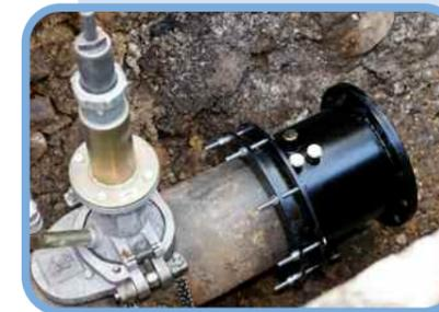
5 Completed V33 ready for connection to new pipe
