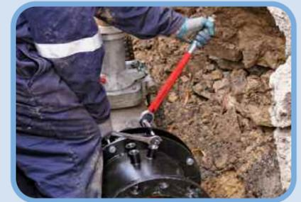
3 Secure the rear seal compression ring
